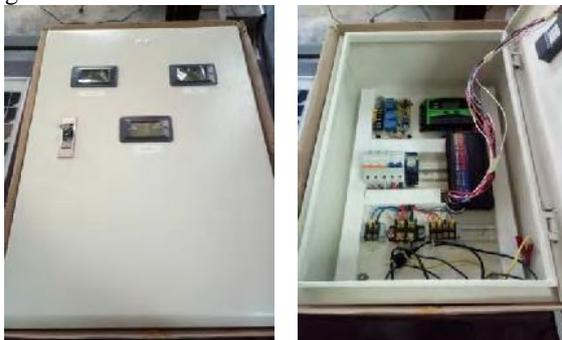
Gambar 9. Panel Auto-Switch Mini PLTS Off-Grid
