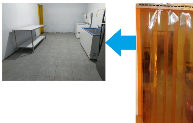
Figure 4. Seal of PVC plastic curtain between space production
